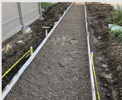
Figure 5 – 25 mm Granular A placement
