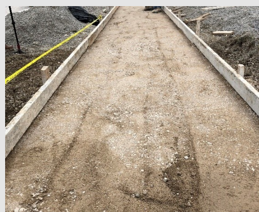
Figure 7 – Subgrade compaction continued and almost ready for concrete
