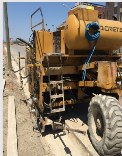
Figure 10 – Concrete curb slip-form paving
