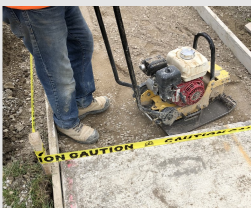
Figure 6 – Subgrade compaction using a vibratory plate compactor
