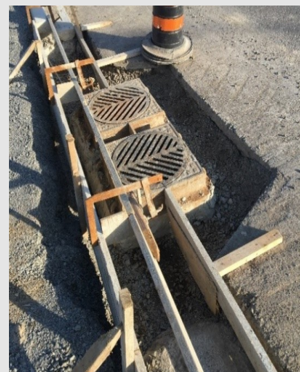
Figure 11 – Hand-curb form set-up around utilities
