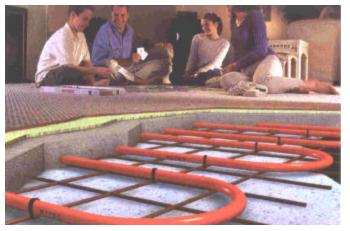
control systems, in conjunction with the spacing of the infloor tubing is used to heat individual rooms within the house to levels set by a thermostat within the room.
