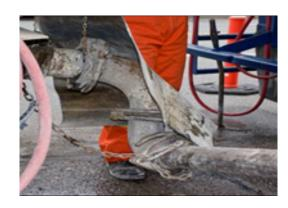
Other areas of concern, include all rigid pipe connectors. These items can undergo wear and the mechanical safety pins installed to prevent the connectors from opening, can unintentionally be knocked out by adjacent construction activities.
