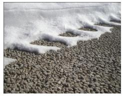
Pervious concrete surface in a cold region
