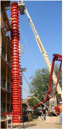
inspected prior to SCC placement. Failure to initially recognize the flowing properties of SCC has resulted in unnecessary concrete placement problems (forgetting to seal around formwork penetrations or thinking that the concrete placement is so far away that you still have time to finish the formwork are common first time mistakes).
