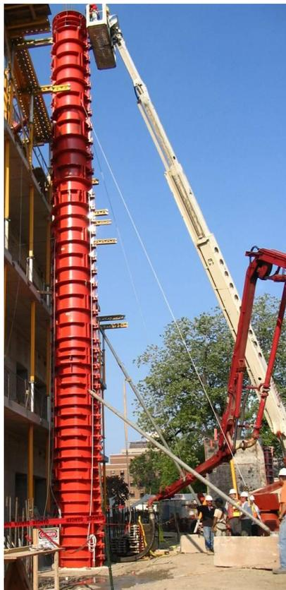
The concrete forming crew must also be aware of the highly flowable nature of the SCC and the fact that while minor gaps in the formwork may result in concrete fins with conventional concrete, SCC can rapidly flow through these gaps resulting in significant material loss and clean-up costs. Also, since this material rapidly seeks to level itself due to gravity, the entire formwork system must be fully constructed and
