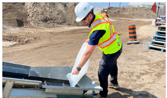
Figure 1: Ice addition to a ready-mix truck
