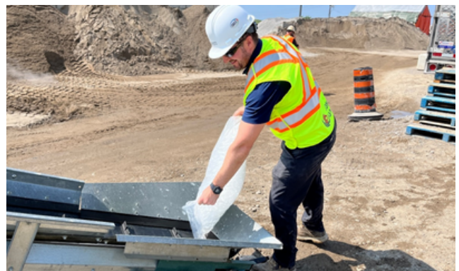
Figure 1: Ice addition to a ready-mix truck
